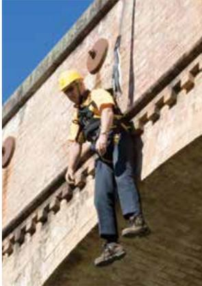
**2** Rescue Pole being used connect to hook to rear of harness
